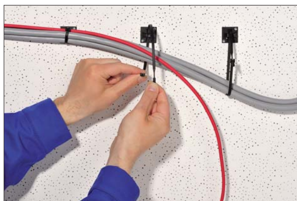
Without additional effort only Q-ties can be used for temporary and final cable bundling.
